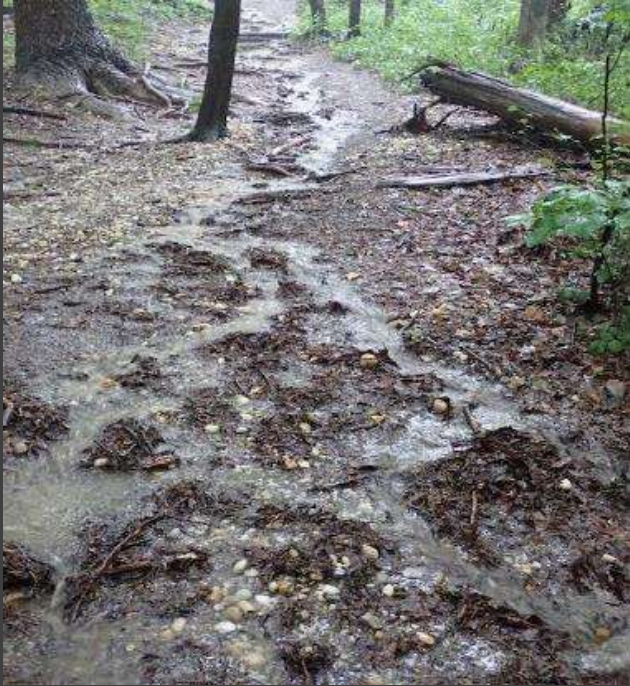
Foot paths need maintenance to slow, divert and absorb runoff.
