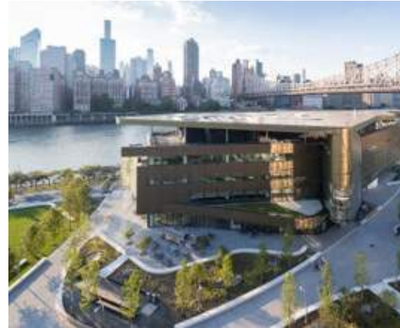
Low carbon buildings with on-site renewables
