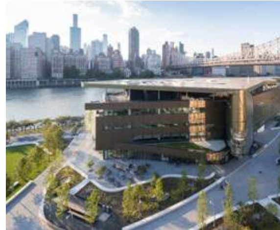
Low carbon buildings with on-site renewables
