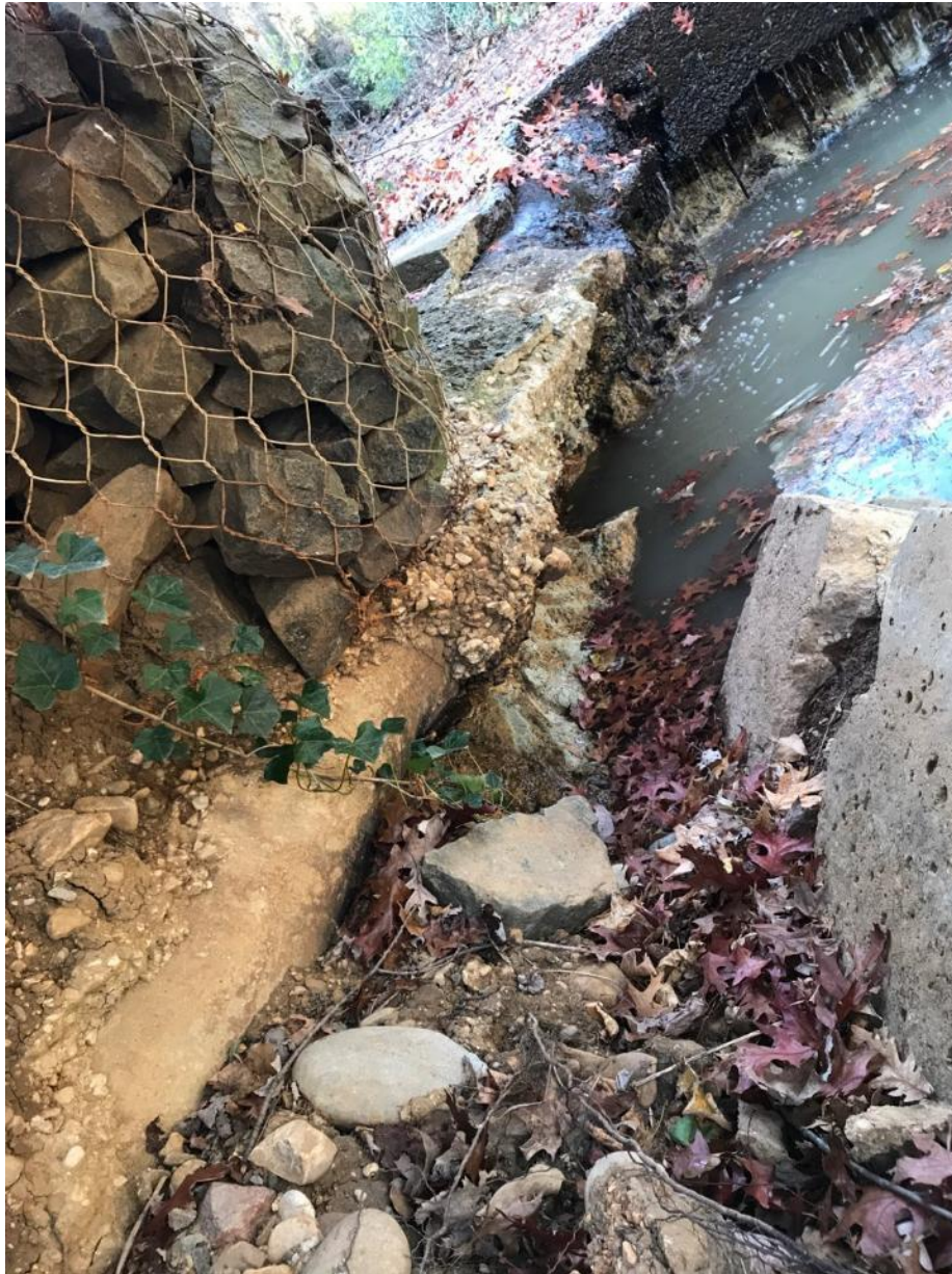
Figure 4-20: Exposed RCP Sewer 00709SEWP beneath pedestrian bridge in Tributary to Taylor Run
