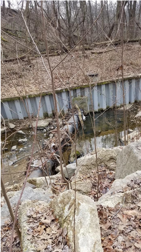
Figure 4-10: Exposed Sewer Crossing 009478SEWP with supports
