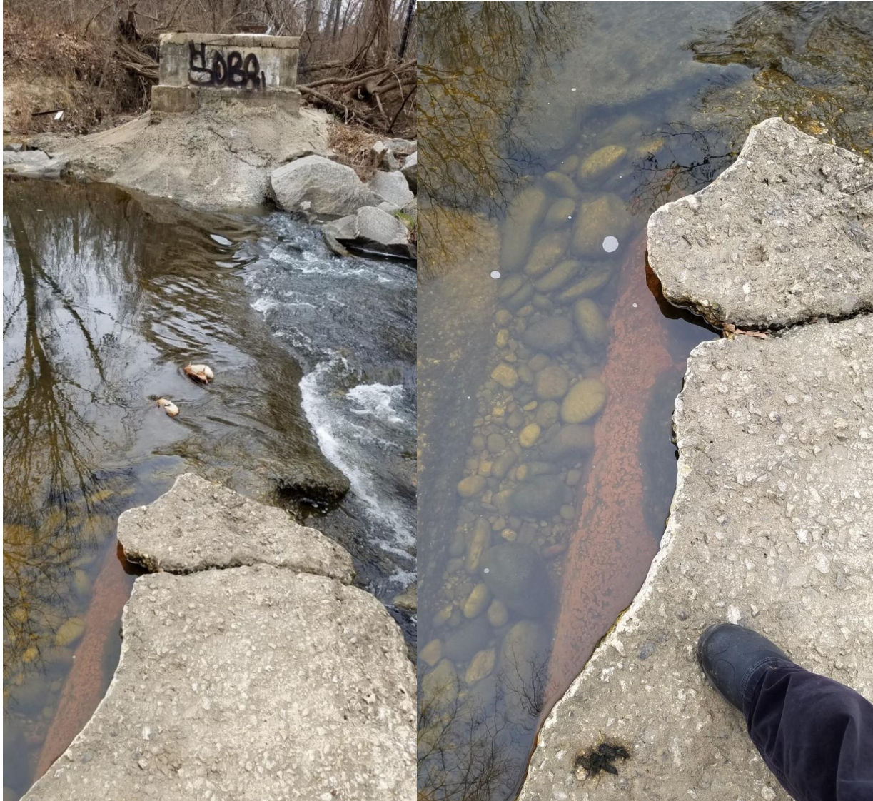
Figure 4-2: Looking East along the Crossing (002618SEWP) with Close-up
