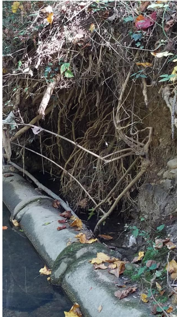
Figure 4-6: Exposed Sewer Segments in Lucky Run along eroded streambank 009524SEWP
