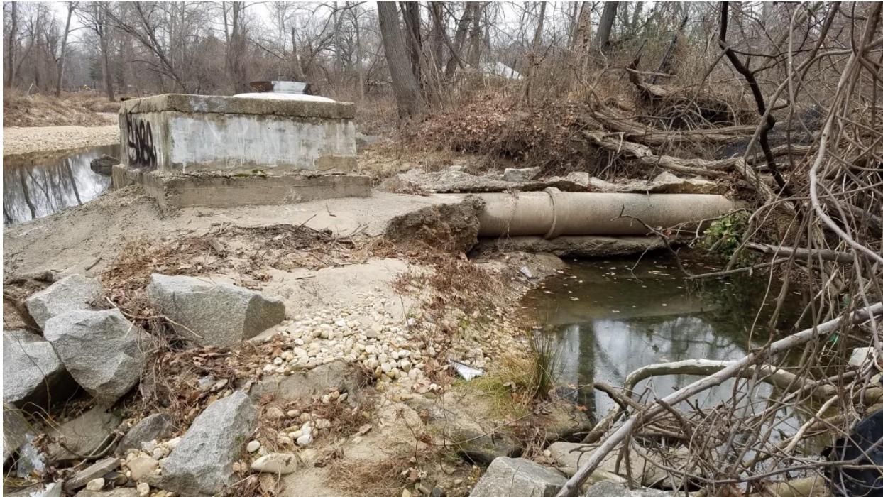
Figure 4-4: Looking West (downstream on tributary) along exposed 002639SEWP towards 002476SSMH
