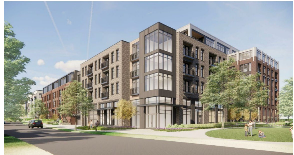
The Heritage at Old Town, the first project to use the RMF Zone
