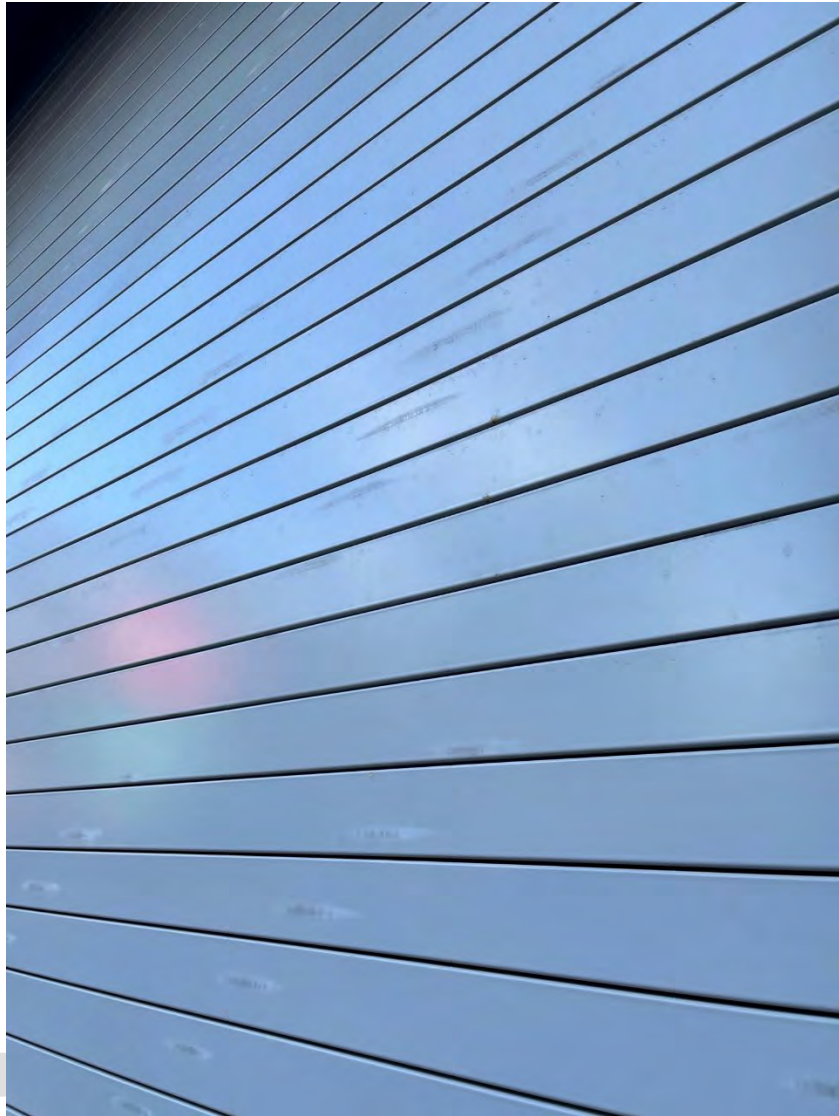
Image: Loading door close up
