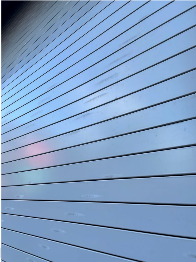
Image: Loading door close up
