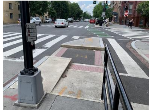
Figure 8: Accessible Push Button with Audible Cues at an Island Bus Stop Source: KFH Group
