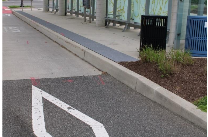
Figure 53: Curb Height Rise for Near-Level Boarding
