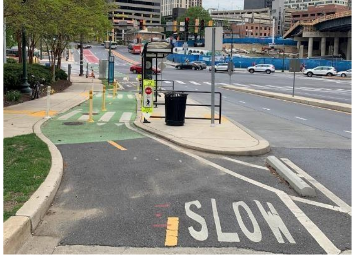
Figure 33: SLOW Bike Lane Pavement Warning at Island Bus Stop
