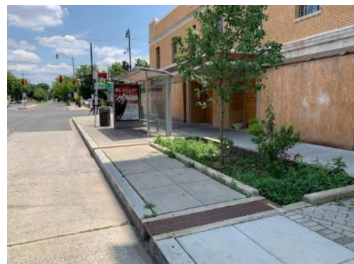
Figure 10: Bioretention Area with ADA Compliant Trench Drain Grates Source: KFH Group
