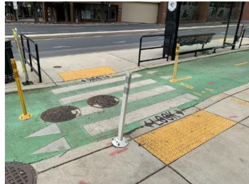
Figure 6: Detectable Warning Surfaces Placed at Bike Lane Pedestrian Crossings
