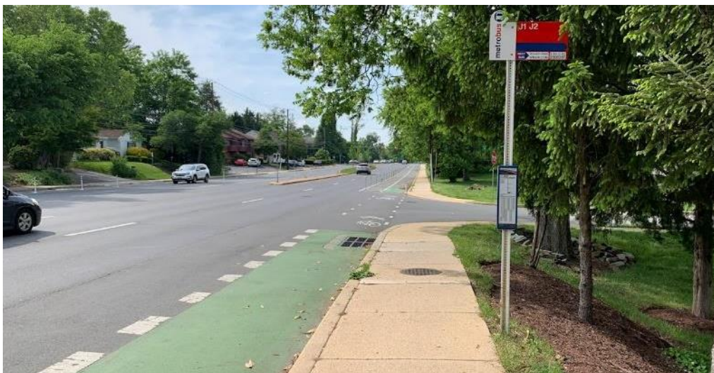
Figure 42: Mixing Bike/Bus Stop with Bike Lane and Roadway Markings
