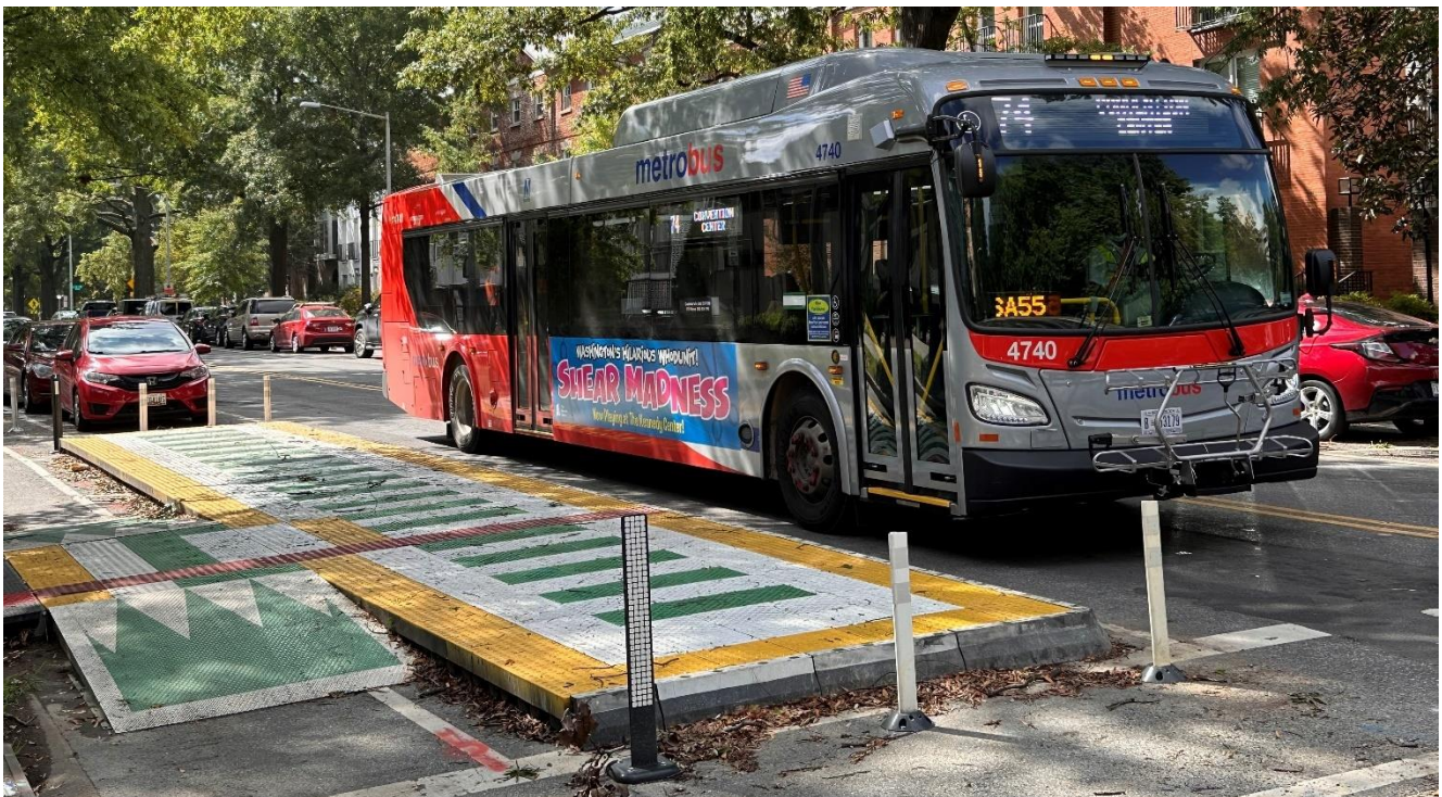
Figure 21: Modular Platform Used for Bus Stop
