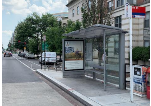
Figure 28: Shelter Used as Barrier to Direct Passengers Towards Crossing
