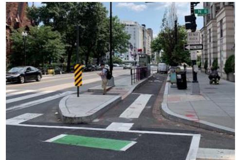
Figure 30: Channelized Bike Lane
