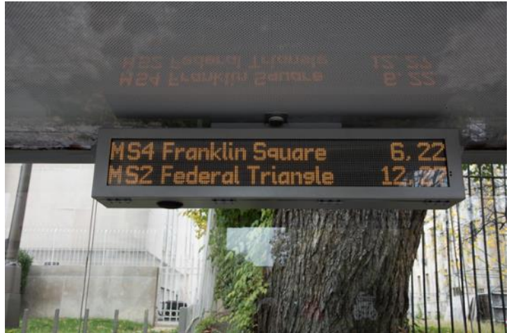
Figure 59: Real-Time Passenger Information Signage
