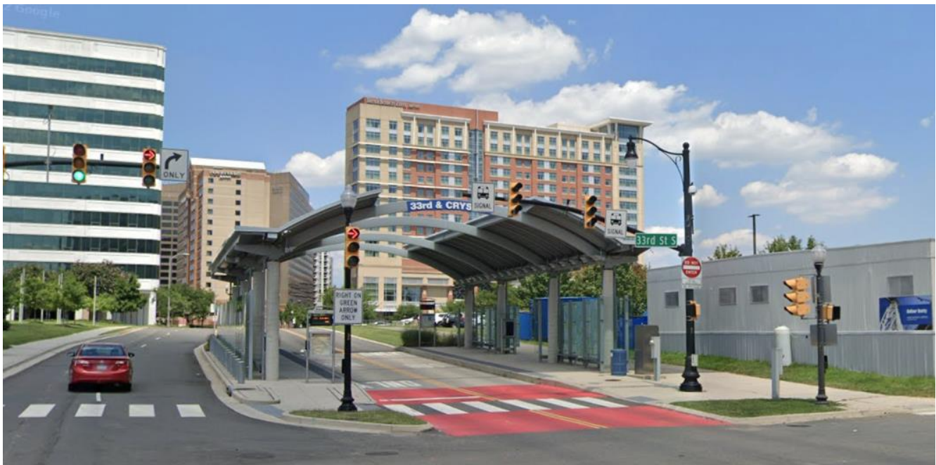
Figure 44: Crystal City Potomac Yard Transitway BRT Bus Stop
