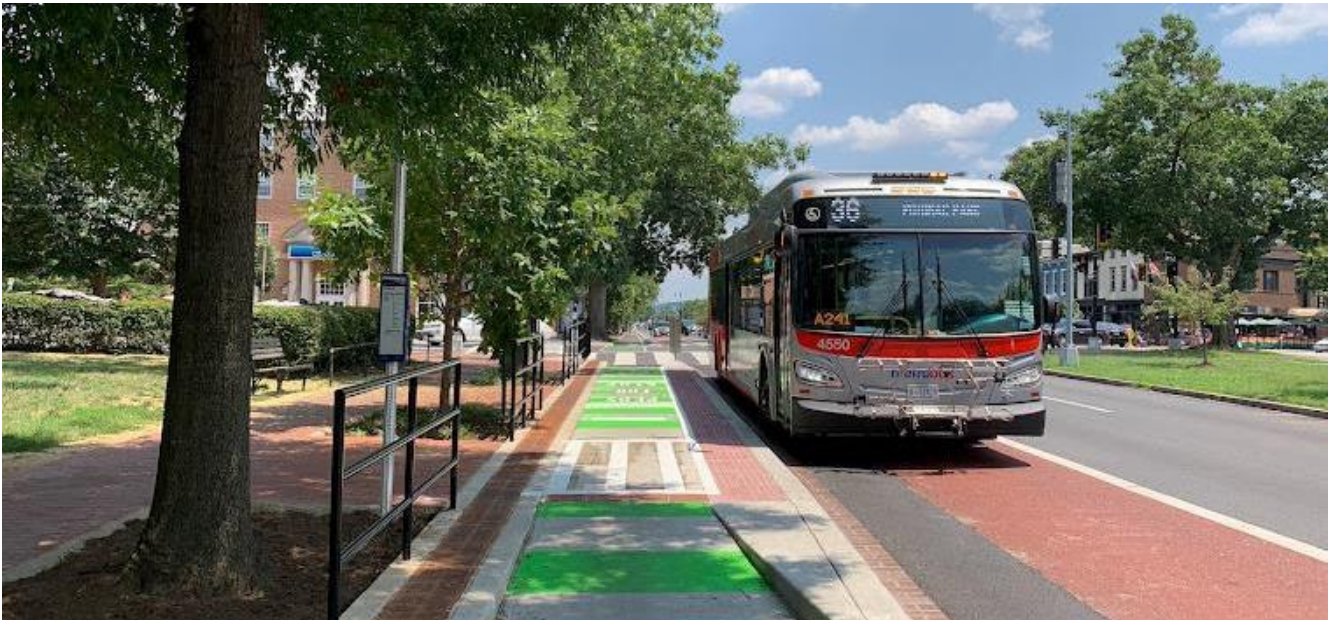
Figure 40: Shared Bus/Bike Stop with Detectable Warning Surfaces and Railing
