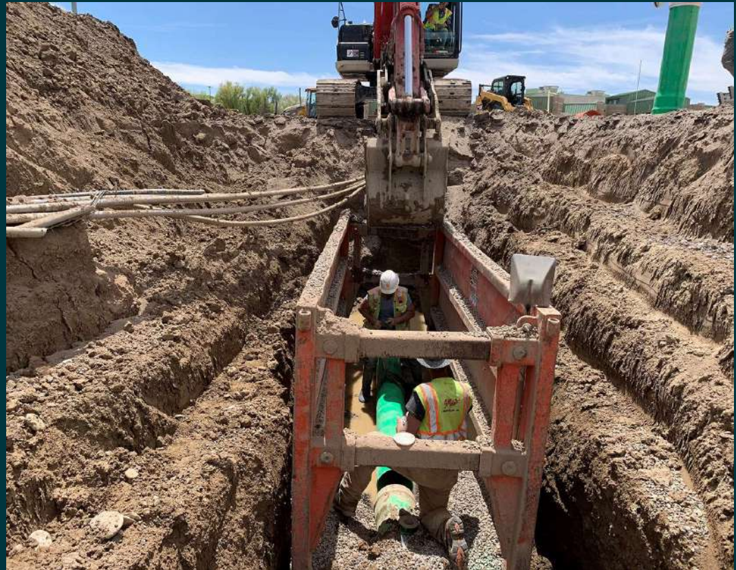
Delta, CO Sewer Realignment Source: Skip Houston Construction
