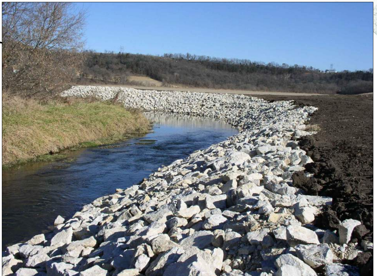
RIPRAP BANK PROTECTION
