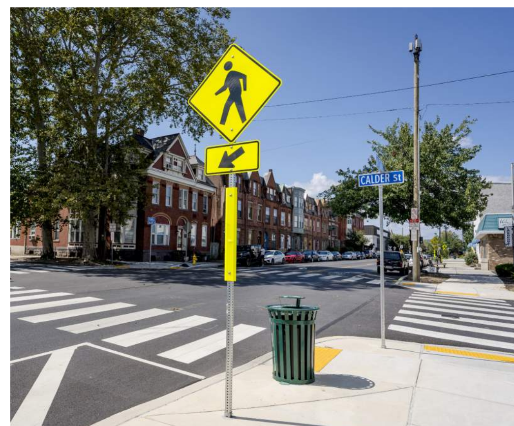
High Visibility Crosswalk / Cruce Peatonal de Alta Visibilidad
