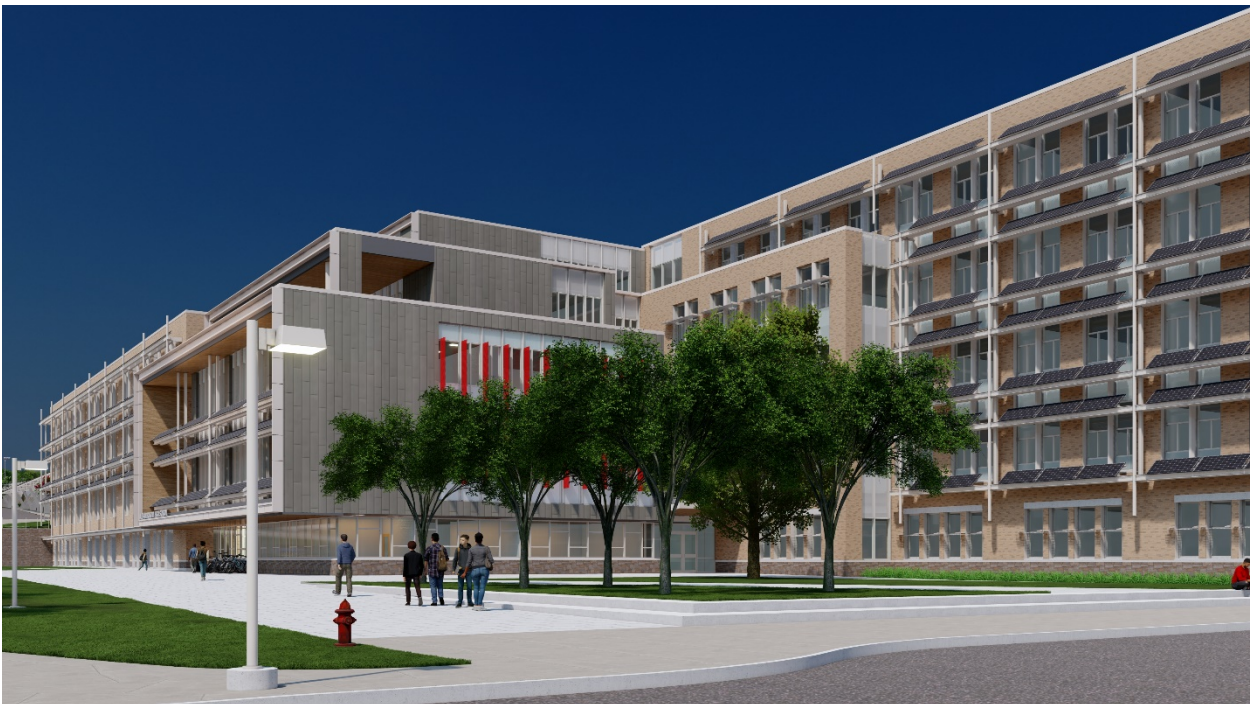
Entry Pavilion from eastern parking lot area (SE corner)
