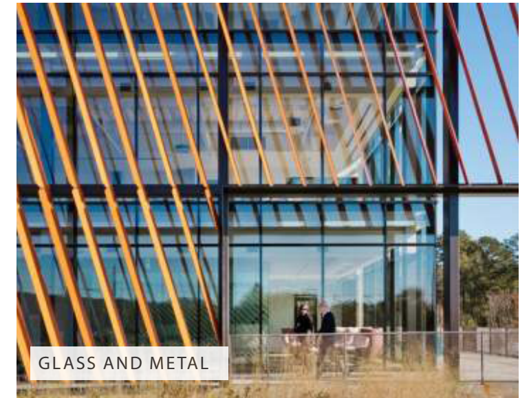
GLASS, METAL PANEL AND TERRA COTTA
