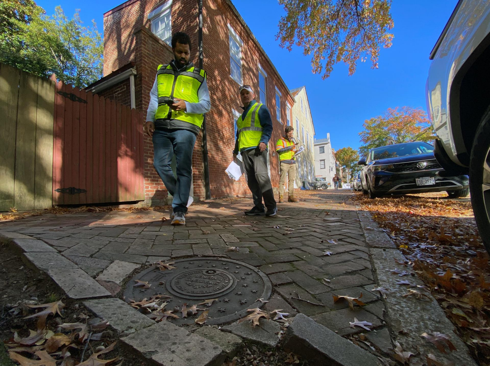
TOP: Engineers with contracting firm Jacobs Engineering map infrastructure on Prince Street for a proposed flood mitigation project. BOTTOM: City engineers Lu Zhang (left) and Jonathan Whiteleather (center) talk with Laura Bendernagel, an engineer from RK&K, as they conduct a site walk on East Abingdon Drive. (City of Alexandria)
