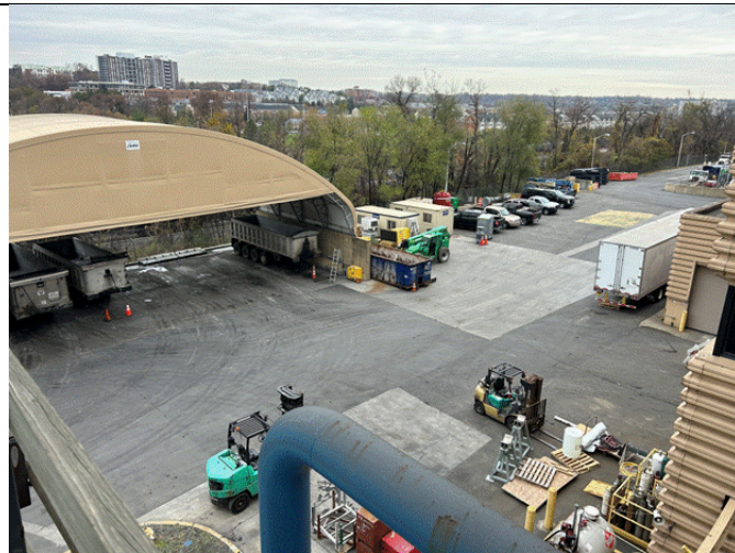
Figure 11: Pavement refurbished on the North side of the Facility.
