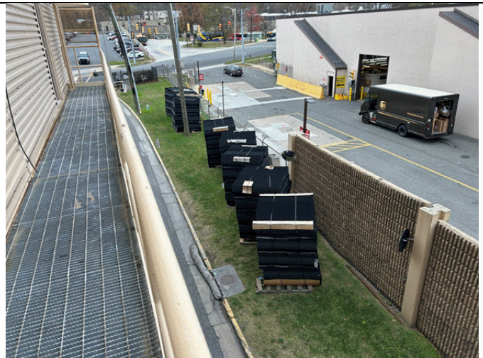
Figure 12: Cooling Tower packing material on-site for replacement.
