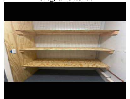
Built shelving for warehouse supply room.
