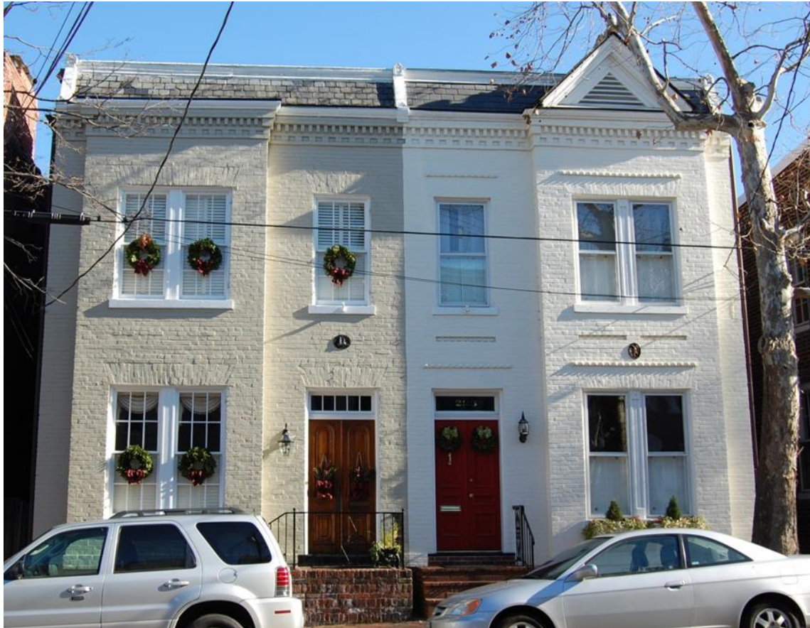
Inappropriate window replacement and Victorian brick ornament removed from house on the left to make it look older than it is.
