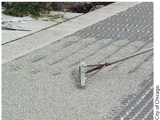
Raking gravel into a Gravelpave2 system.
