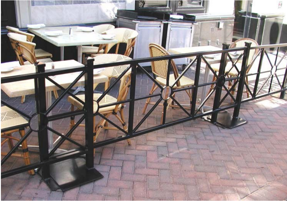
Acceptable sectional fencing design: freestanding
