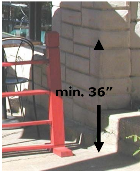
Sectional fencing barrier height must be at least 36" and no taller than 48 inches
