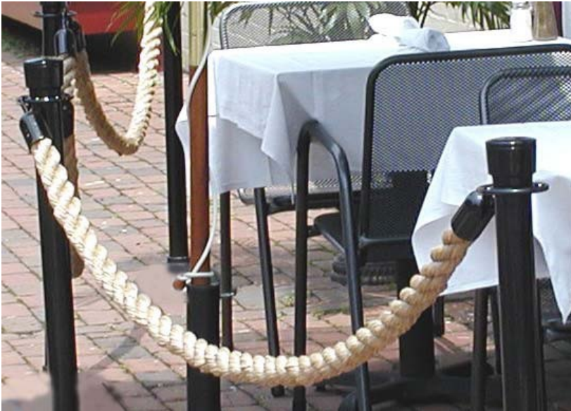
Rope or chain barrier must have a minimum diameter of 1 inch
