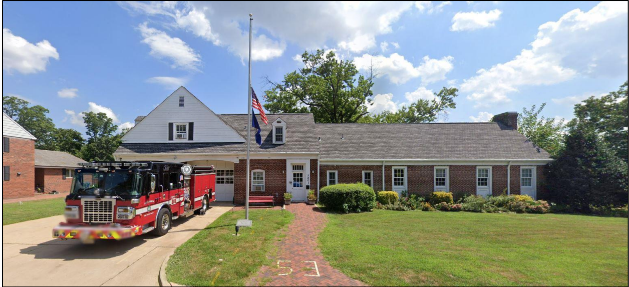
Figure 23. Firehouse at 2801 Cameron Mills Rd., Alexandria (Google 2022).
