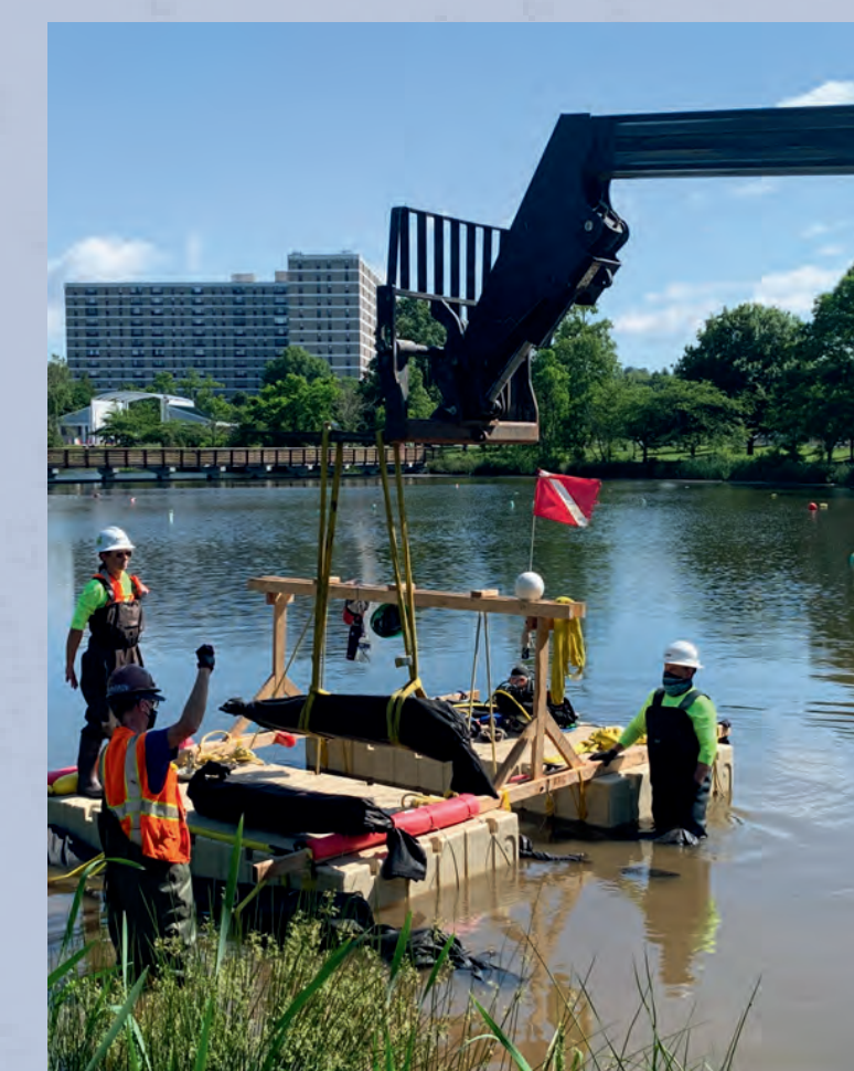
Loading timbers onto floating dock
