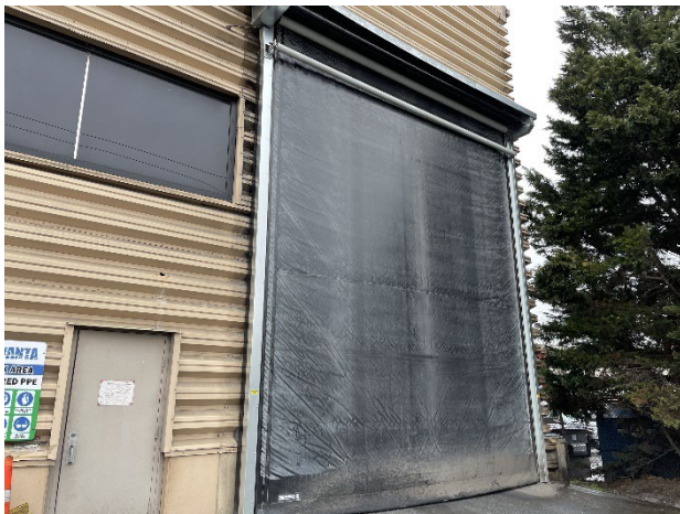
Photo: New high-speed roll-up door installed for trucks exiting tipping floor.
