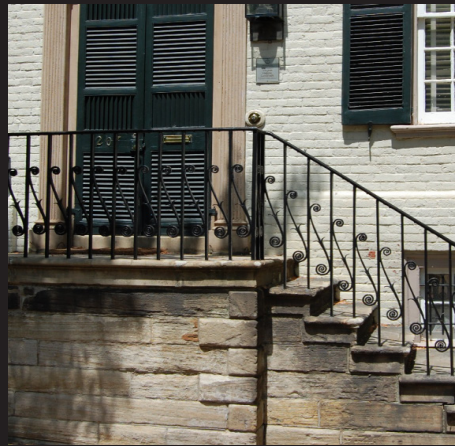
Example of historically appropriate stone steps, iron handrail and guardrail on a Georgian style residence.
