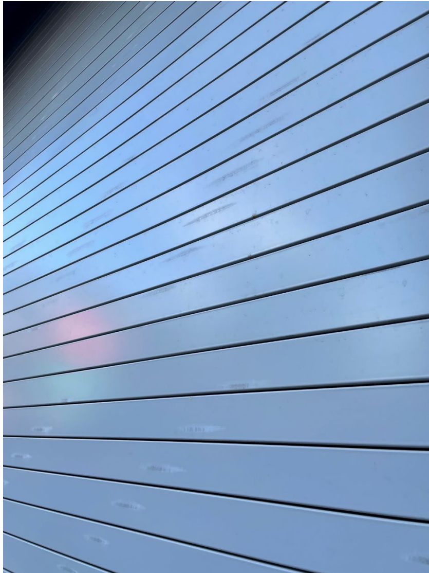
Image: Loading door close up
