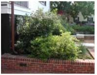
Stormwater planter connected to roof downspout
