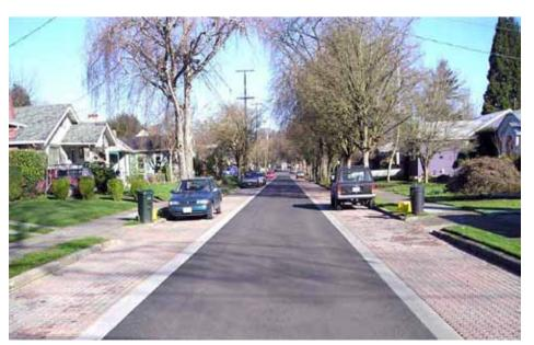
Permeable pavers used in the on-street parking area of the roadway
