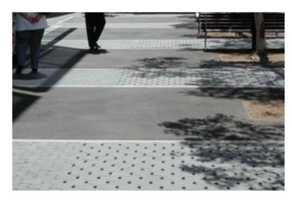
Examples of paving materials used in combination. Above, castin-place concrete, stone and recycled rubber; below, asphalt and permeable pavers
