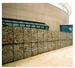
Stone and gabion clad concrete wall
