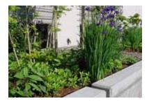
Stormwater planter with slotted curb
