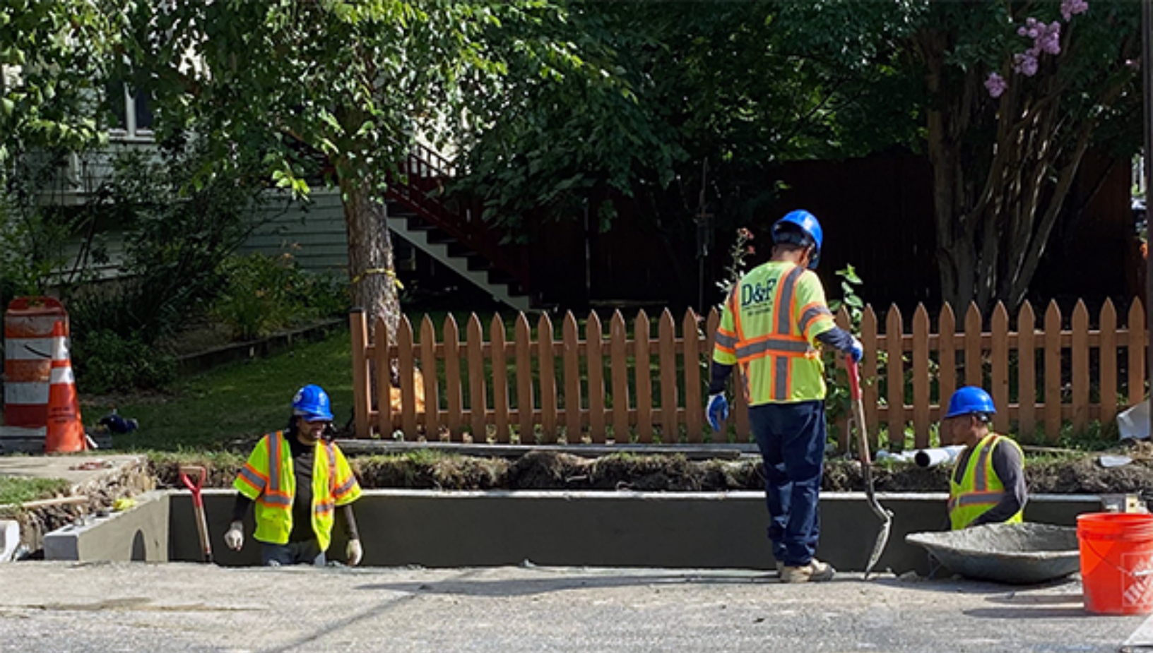
Contractors from D&F Construction break ground to install larger storm drain inlets on West Del Ray Avenue on July 25. (City of Alexandria)
