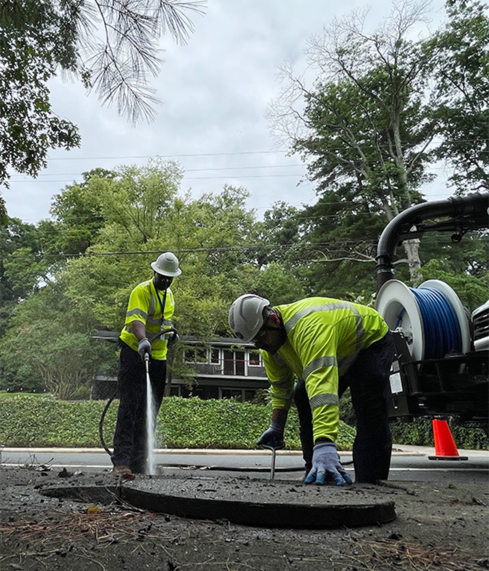
Public Works Division employees Raymond Monk (left) and Danny Rivera (right) remove debris clogged in a storm drain on Polk Avenue on July 19. (City of Alexandria)
