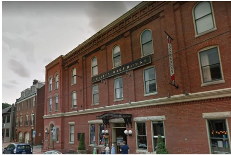
Crilley Warehouse Building in 2018
