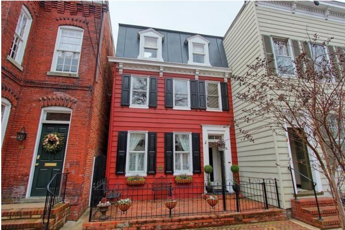
The Evans Dulaney Home at 806 Duke Street, Alexandria, VA. This was the family residence in the early 20 th century.
