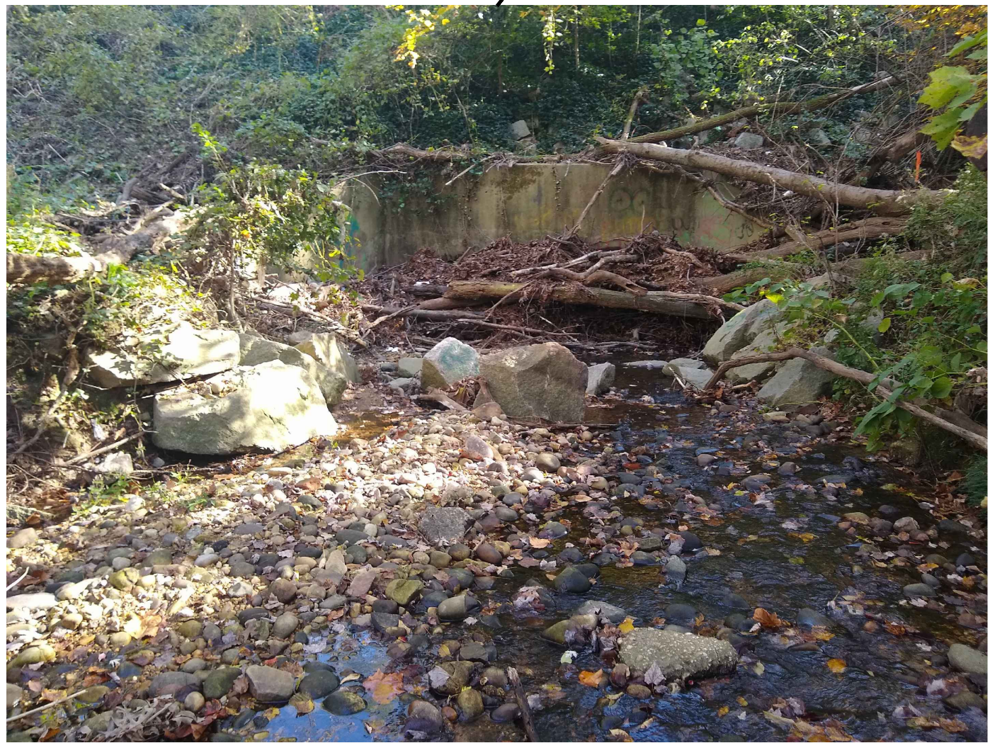
EXISTING DEBRIS BLOCKAGE
