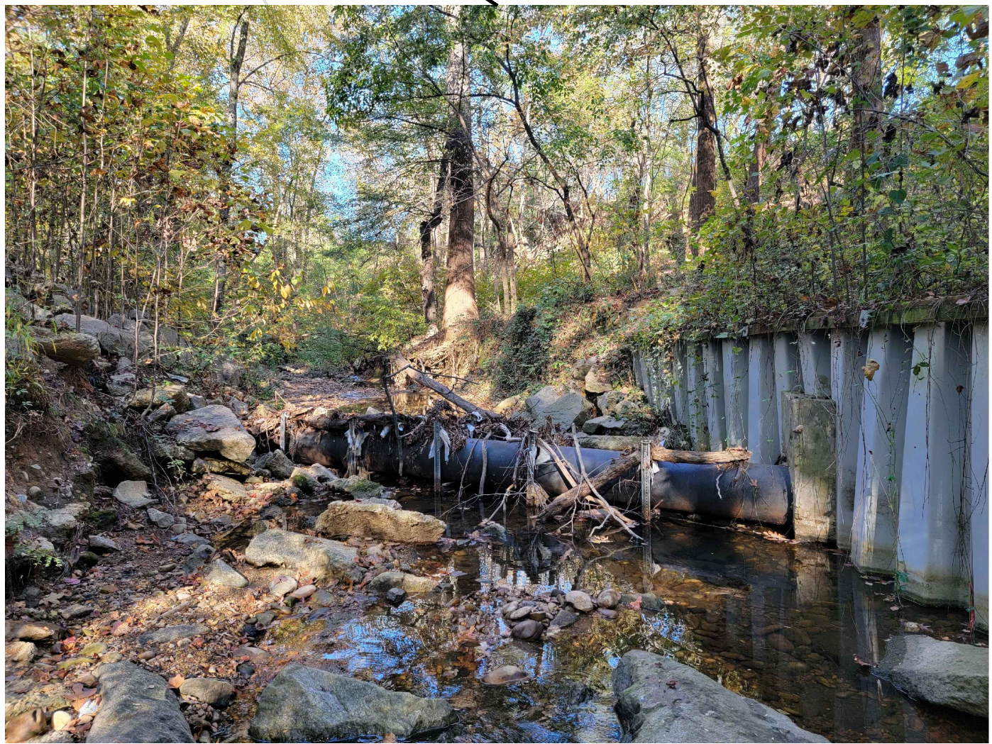
EXISTING EXPOSED SANITARY SEWER CROSSING AND COLLAPSING SHEET PILE WALL
