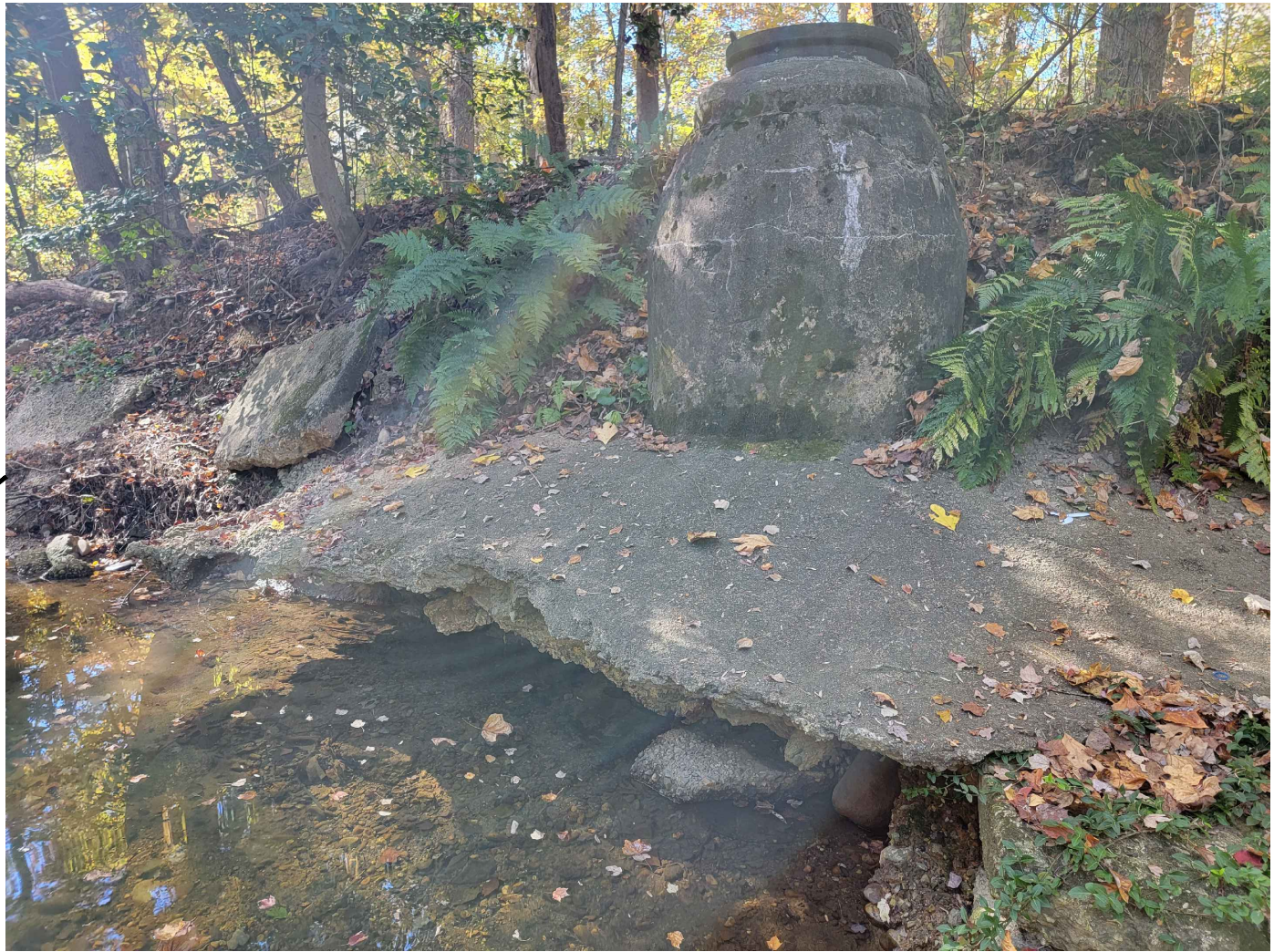
EXISTING UNSTABLE MANHOLE UNDERMINED BY EROSION
