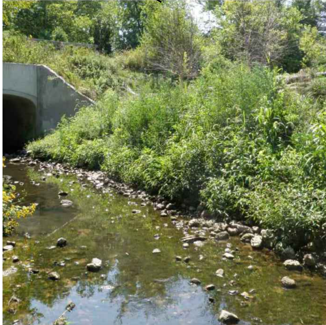
VEGETATED WALL EXAMPLE (1-2 YEARS POST CONSTRUCTION)
