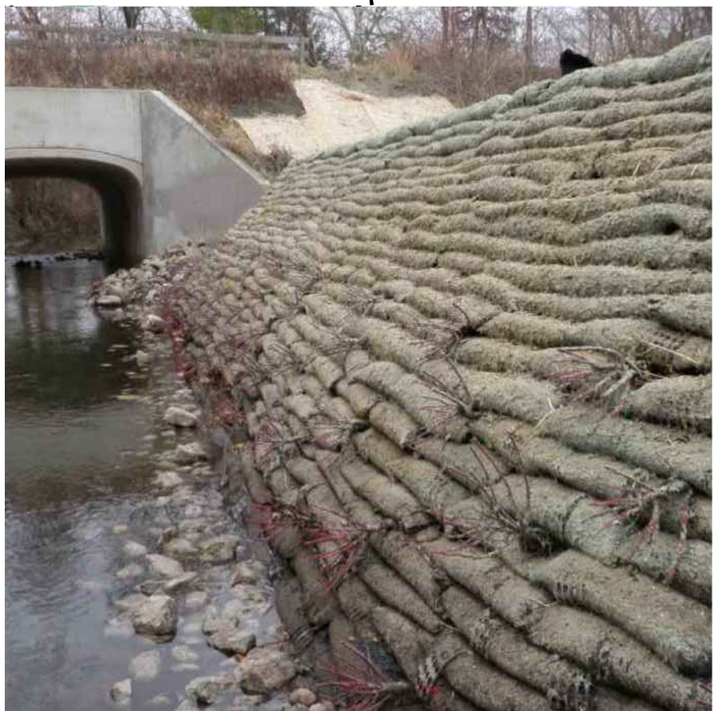
VEGETATED WALL EXAMPLE (RECENTLY INSTALLED)
