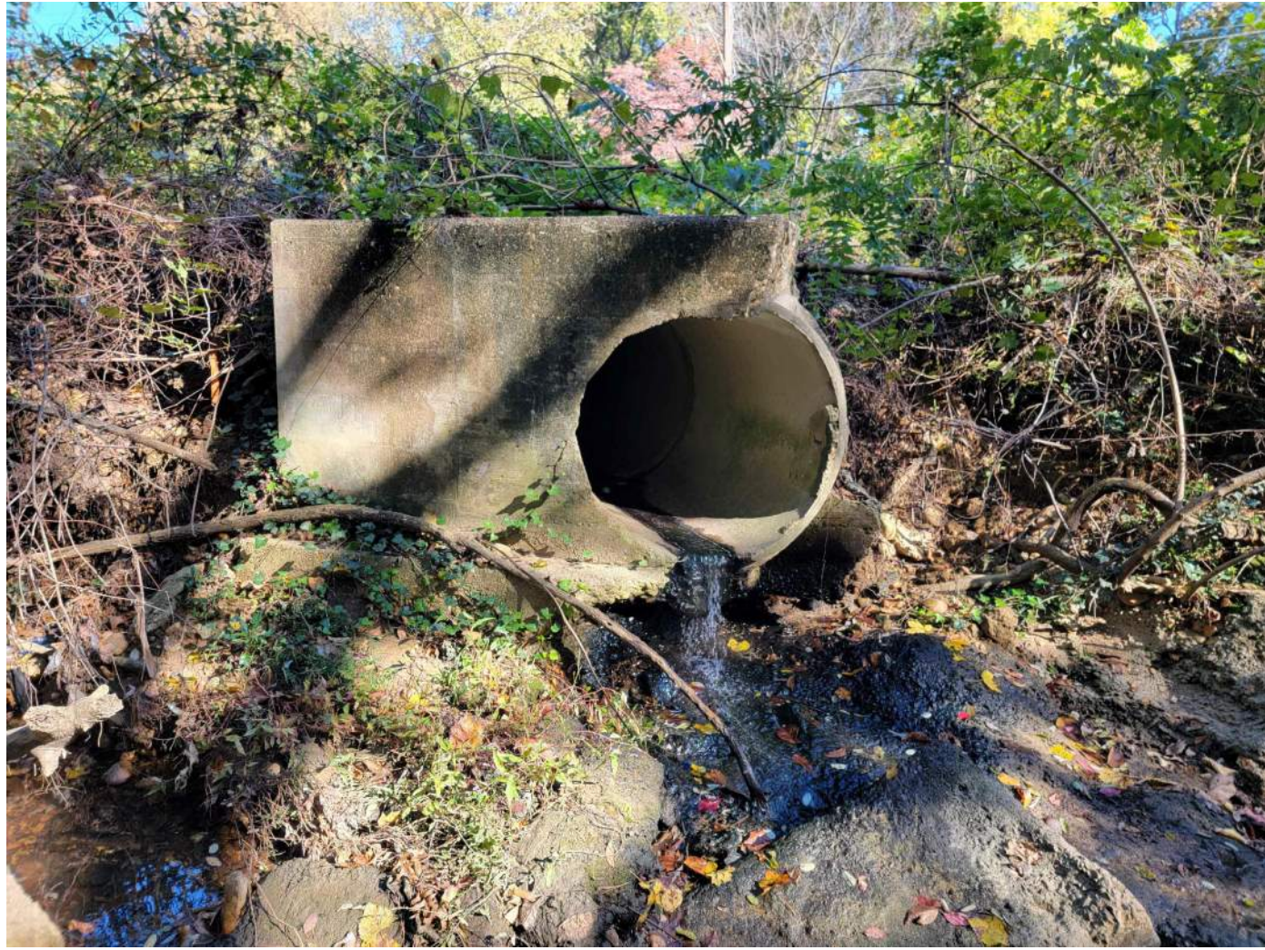
BROKEN CONCRETE HEADWALL
