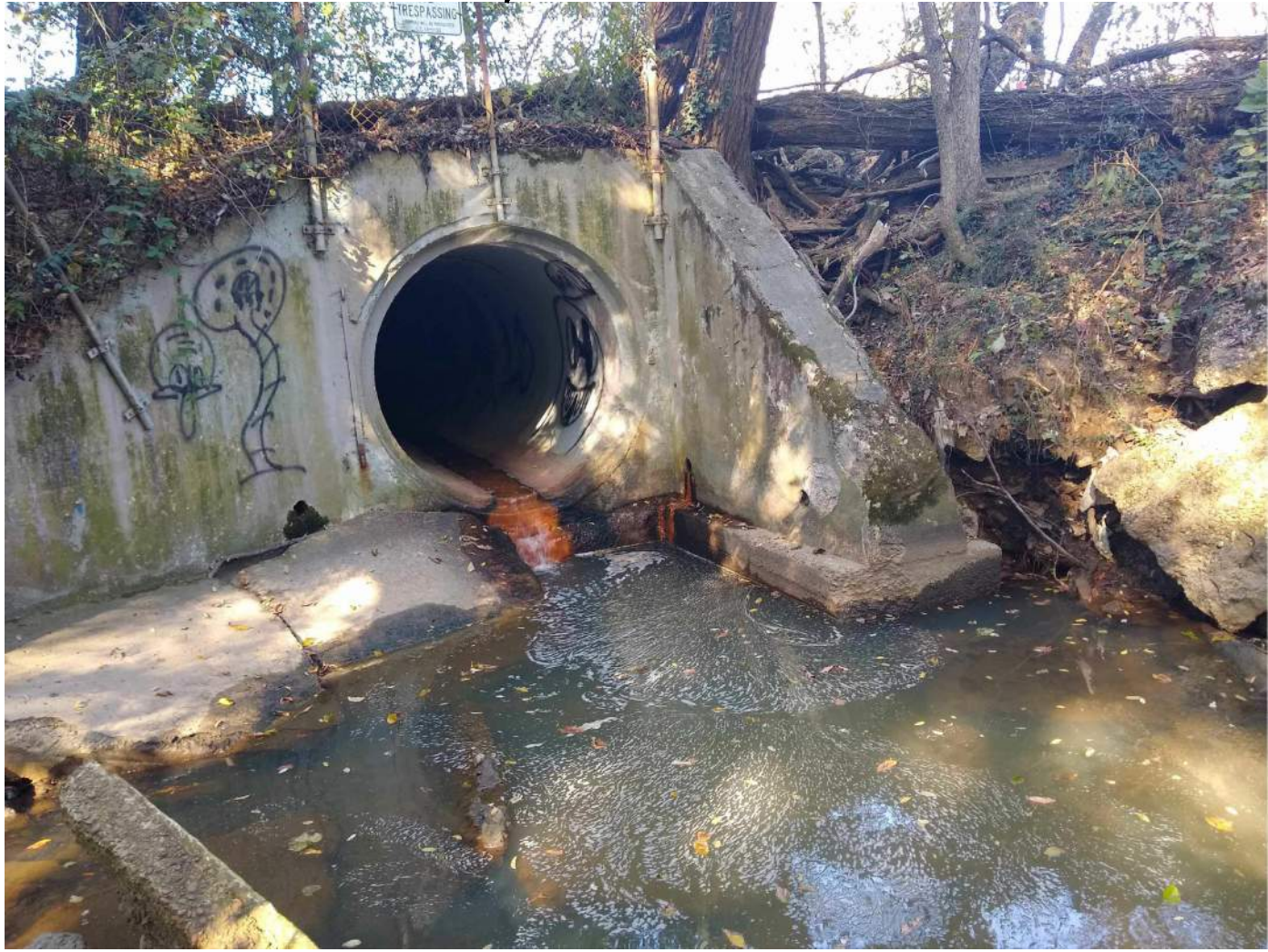
EROSION ADJACENT TO CONCRETE HEADWALL
