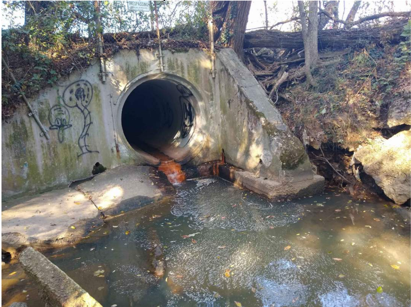
EROSION ADJACENT TO CONCRETE HEADWALL
