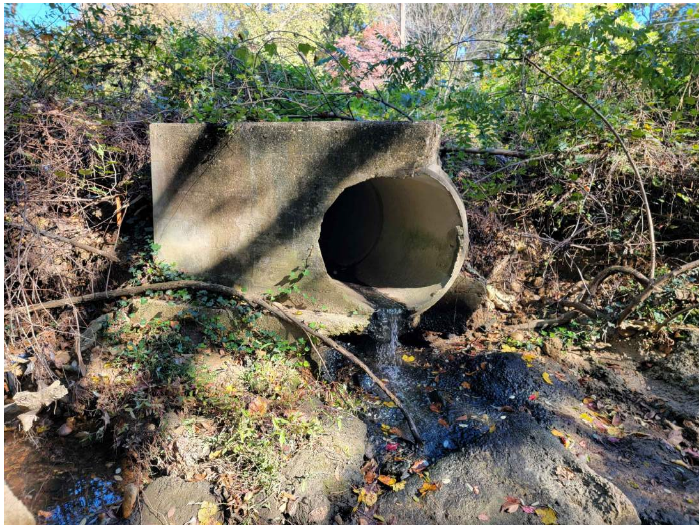
BROKEN CONCRETE HEADWALL
