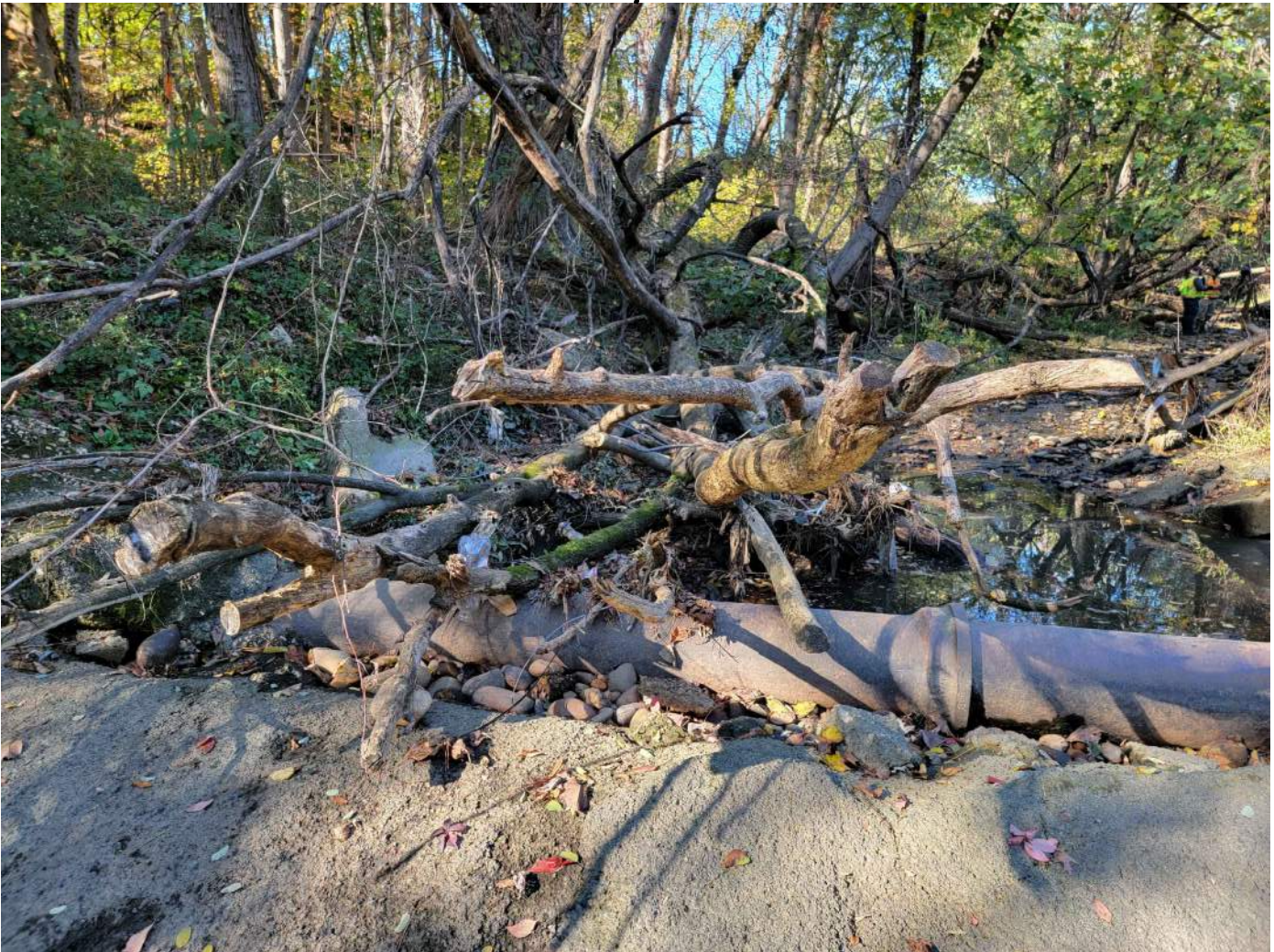
WOODY DEBRIS ACROSS UNSTABLE EXPOSED SANITARY SEWER CROSSING
