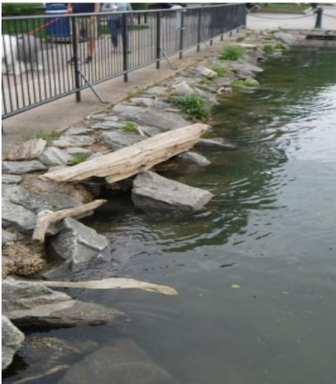
Photo 7 - Waste Concrete and Boulders
