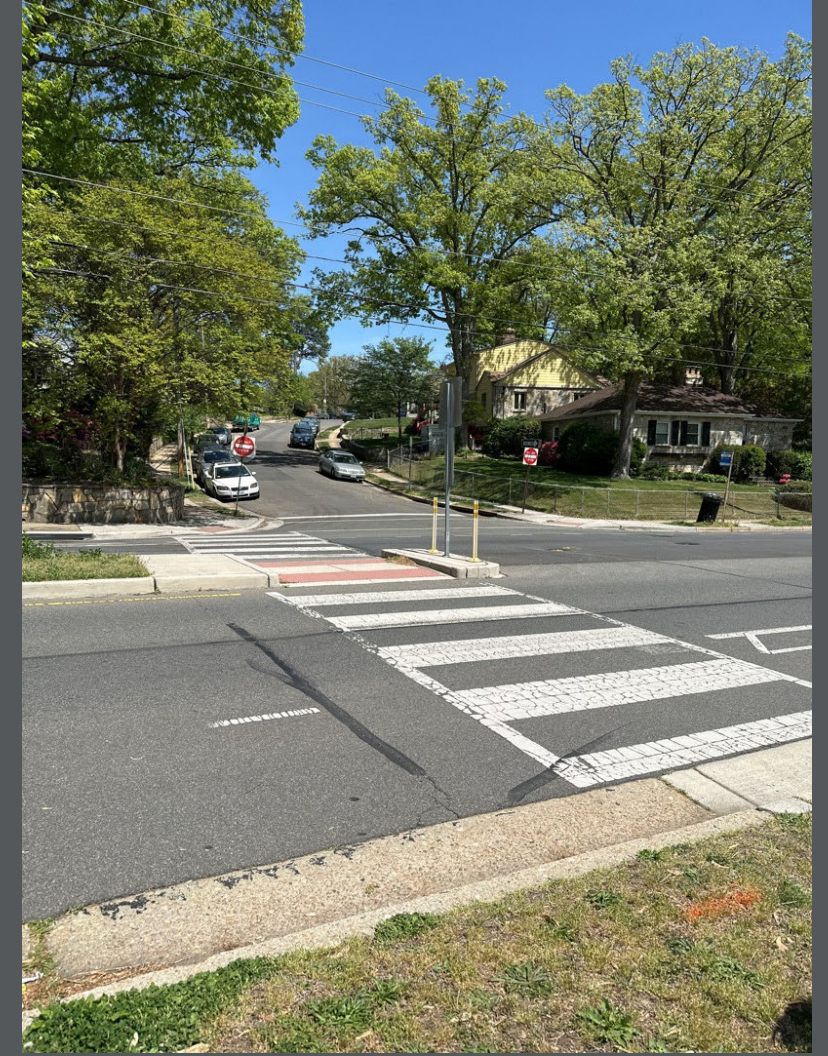
Quincy Street and King Street. There is a signed and marked crossing.
