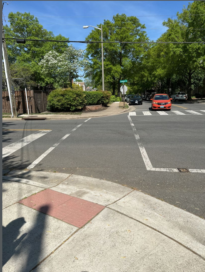
Intersection of Dogwood Drive and Kenwood Avenue. This is a 4-way stop controlled intersection, with marked crosswalks and detectable warning surfaces on 2/4 curb ramps.
