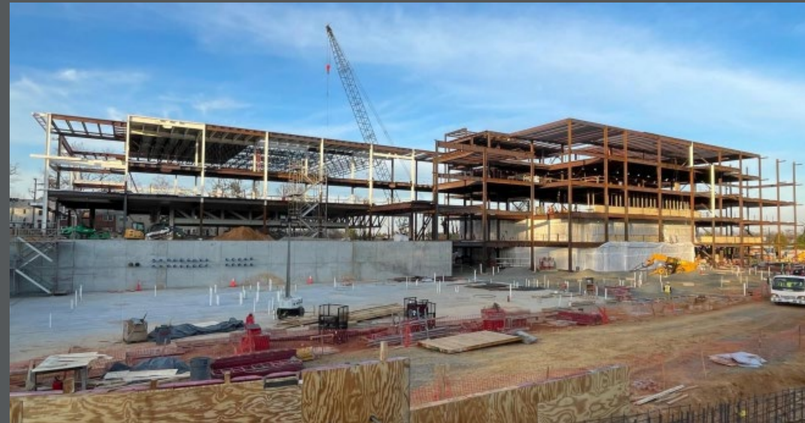
Construction status as of January 2023
