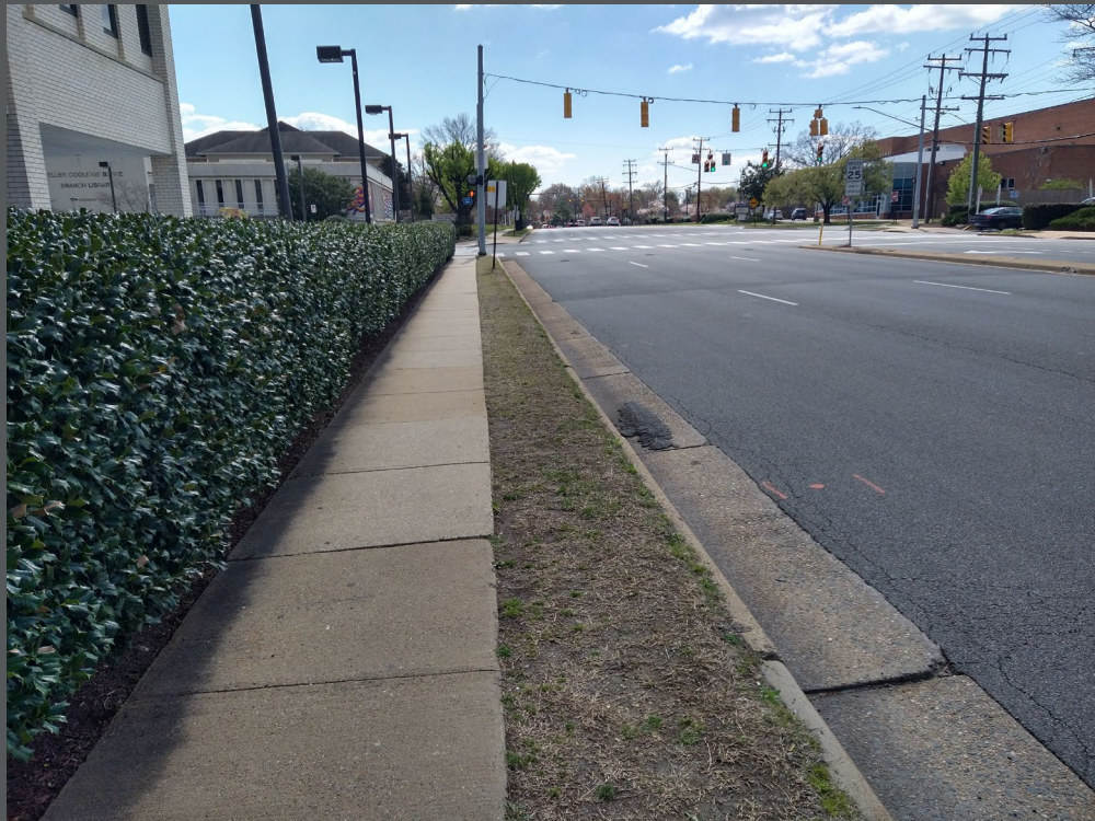
Much of the sidewalk along Seminary Road between the I-395 overpass and the school (in upper right of image) not only has very little buffer from speeding traffic but is also lined with a tall hedge that obstructs 1/8 to 1/4 of its width.
