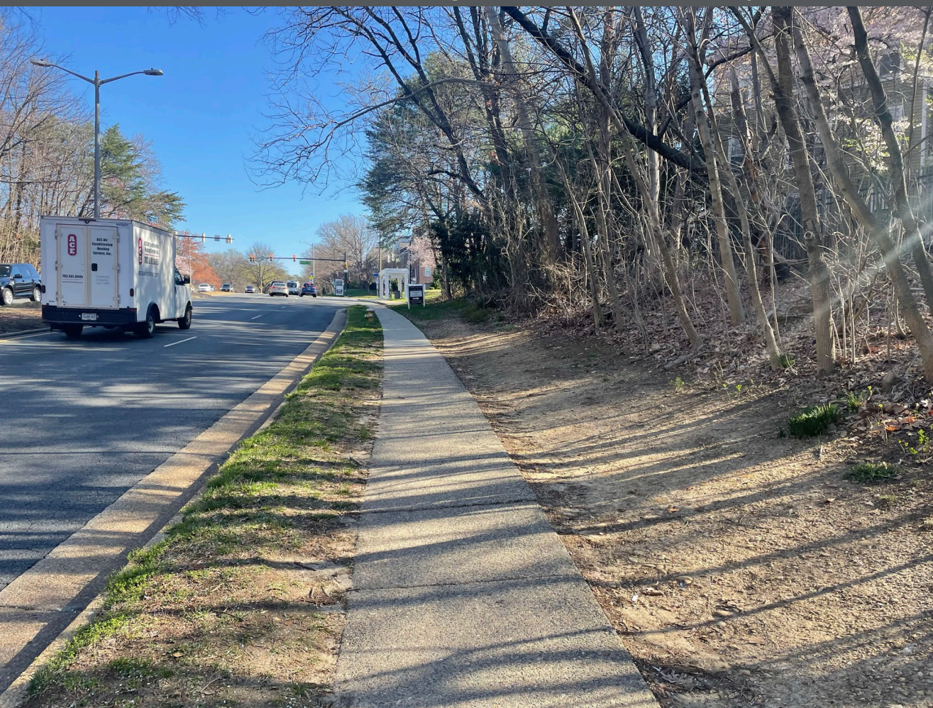
Narrow sidewalk on N Beauregard Street near Rayburn Avenue
