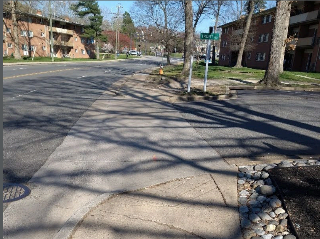
Many apartment building accessways from Sanger Avenue (above) and Roanoke Avenue (above right) aren't clearly defined as streets or driveways. Most, even those like Trent Court (above), which have street signs posted and concrete across their (pavement-level) driveway entrances, do not have marked crosswalks, and curb ramps (if any) have no detectable warning surface.
