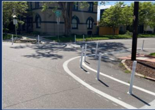
Curb Radii Tightening
