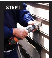
Carefully remove a 2 foot by 2 foot portion of the surface siding.
