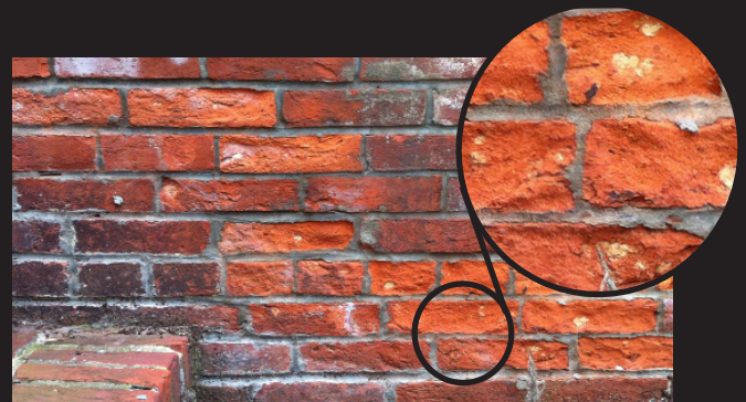
In this example, repointing with a Portland cement mortar has irreversibly damaged the historic brick, causing spalling. Spalling is when the hard-fired face of the brick breaks off due to an impermeable mortar joint.
