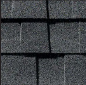
^ ARCHITECTURAL GRADE ASPHALT 20TH - 21ST CENTURY
