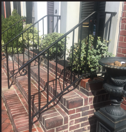
Example of inappropriate modern brick stoop and iron handrail on an Italianate-style residence.
