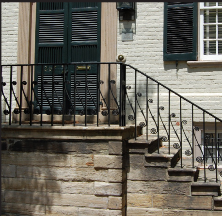
Example of historically appropriate stone steps, iron handrail and guardrail on a Georgian-style residence.
