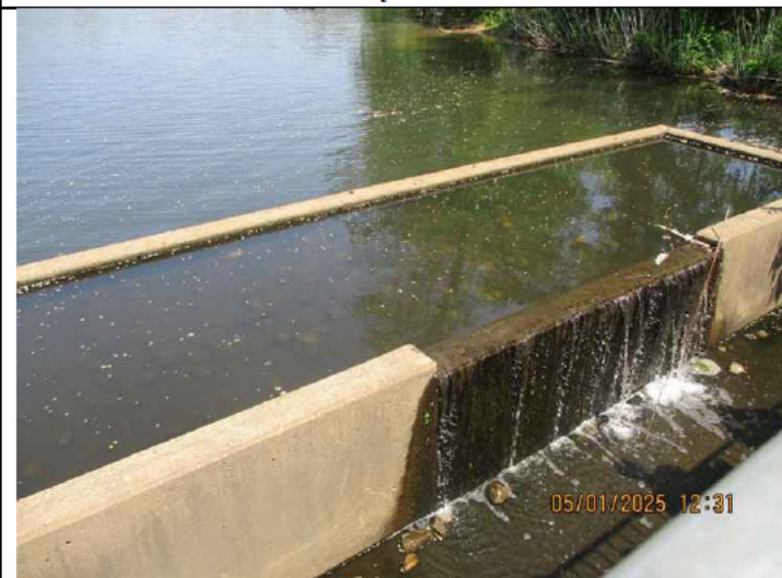
5. Upflow filter at pond outlet structure.
