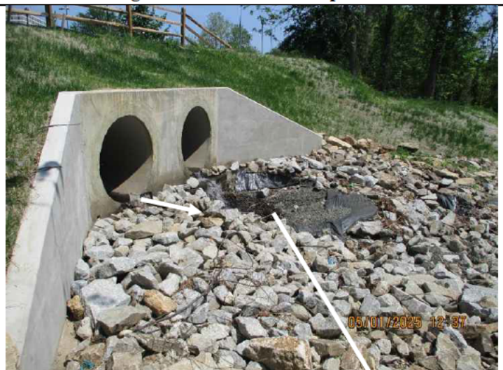
6. Outlet structure showing underlayer exposed at base of the concrete culvert. Observation addressed by
