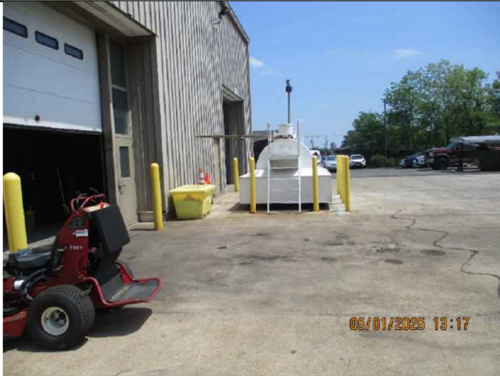
9. 2,000-gallon motor oil and hydraulic oil tank.
