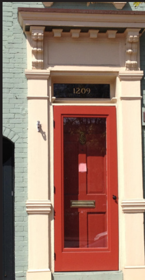
This clear glass storm door is appropriate because it allows the original door to remain visible.
