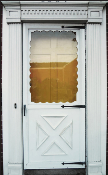
This cross-buck-style metal storm door is inappropriate because it obscures the view of the original door.
