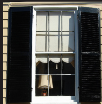
^ 6/6 FEDERAL / GREEK REVIVAL
