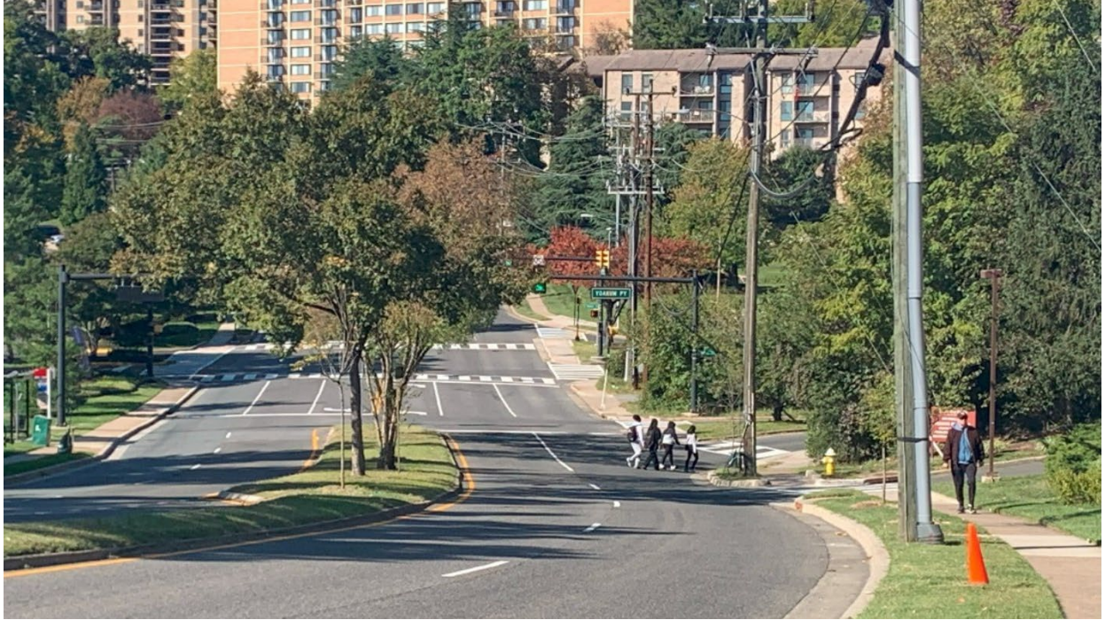
Figure 3. Edsall Road looking west toward Yoakum Parkway.
