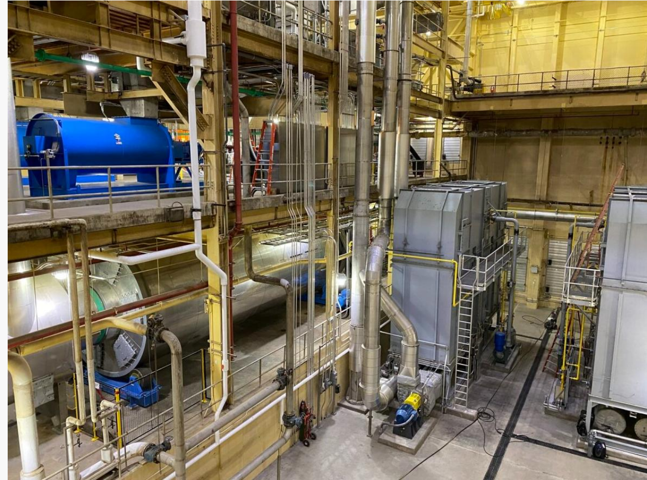
Louisville, KY thermal drying system for biosolids
