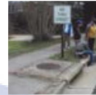
Storm drains are neighborhood entry points to the stormwater system.
