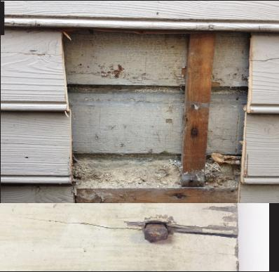
Using clues such as the siding profile and the type of nails used, Staff makes a determination on the age of the siding.
