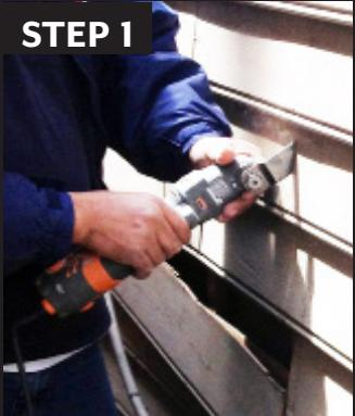
Carefully remove a 2 foot by 2 foot portion of the surface siding.
