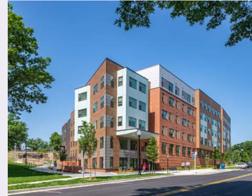
St. James Plaza, an affordable rental community in Beauregard, achieved EarthCraft Platinum, the highest certification in the EarthCraft sustainable building program. The community was made possible by LIHTC funding through a partnership between AHC and the City.
