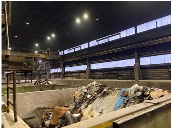
Figure 24: All windows in tipping hall intact
