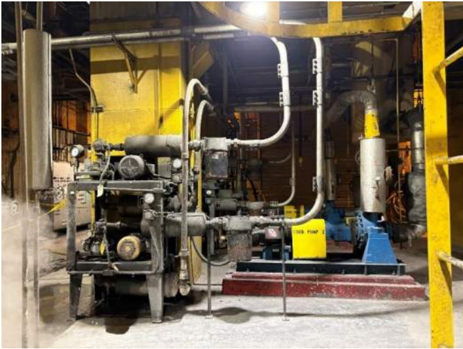
Figure 13: Carbon booster blower system – no issues observed
