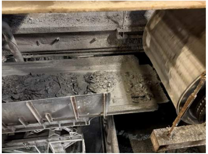
Figure 20: Wet ash prior to ferrous magnet
