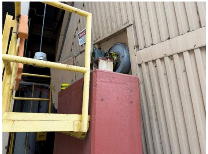
Figure 4: Maintenance observed around ID fan motor
