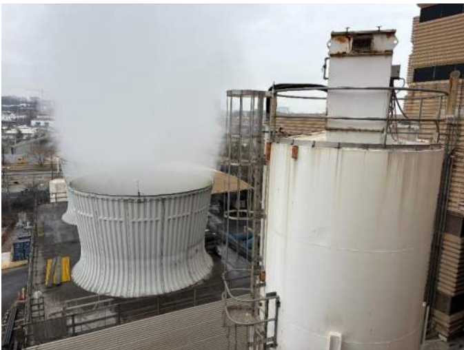
Figure 29: Lime silo baghouse and cooling water tower deck – no issues observed
