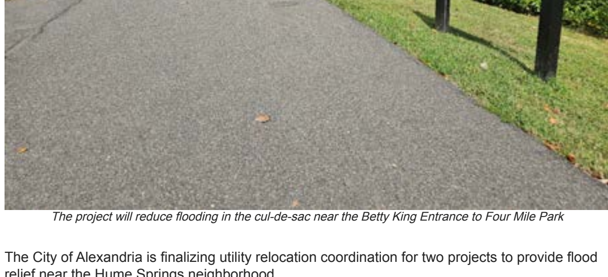
The project will reduce flooding in the cul-de-sac near the Betty King Entrance to Four Mile Park.
